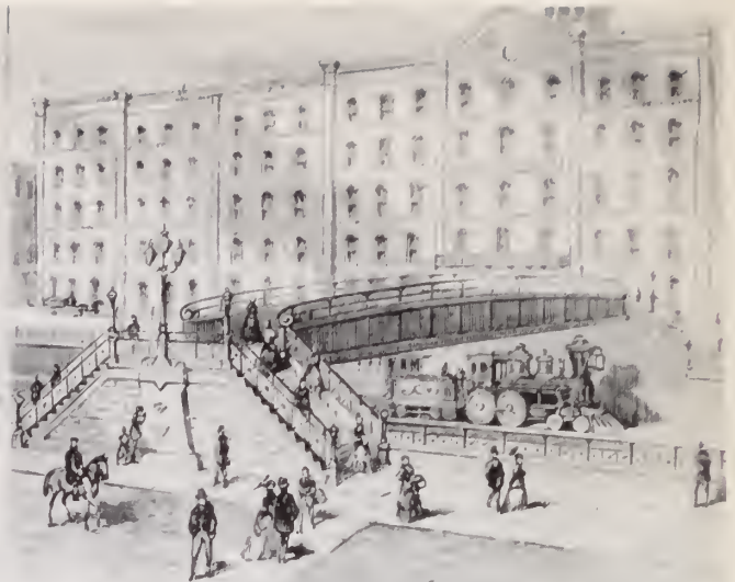
ELEVATED WALK FOR FOOT PASSENGERS BETWEEN 52D AND 53D STREETS.
